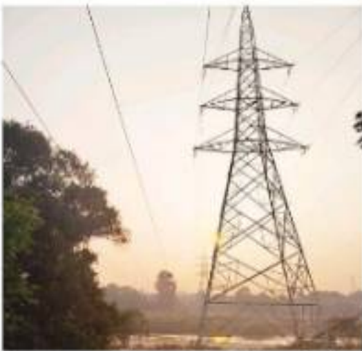
This unit draws supply from two feeders namely Bus stand feeder and medical feeder, providing 24-hour power availability to critical healthcare facilities. The major benefit of installing the RMU is that if any breakdown occurs in one feeder, still power can be supplied across
